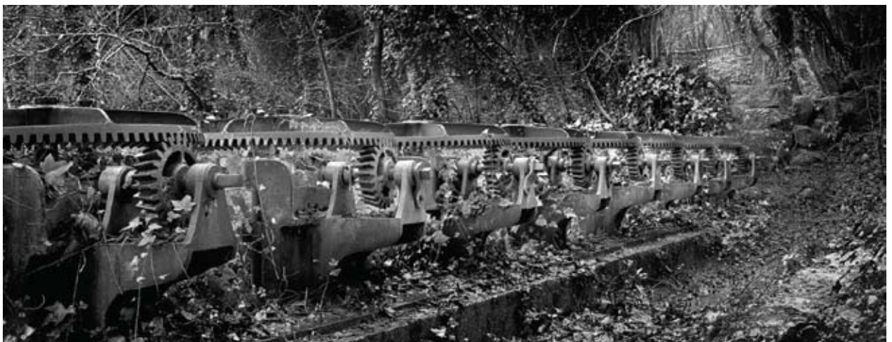
The Old Sluice Gate Clareville Water Works, County Limerick.
